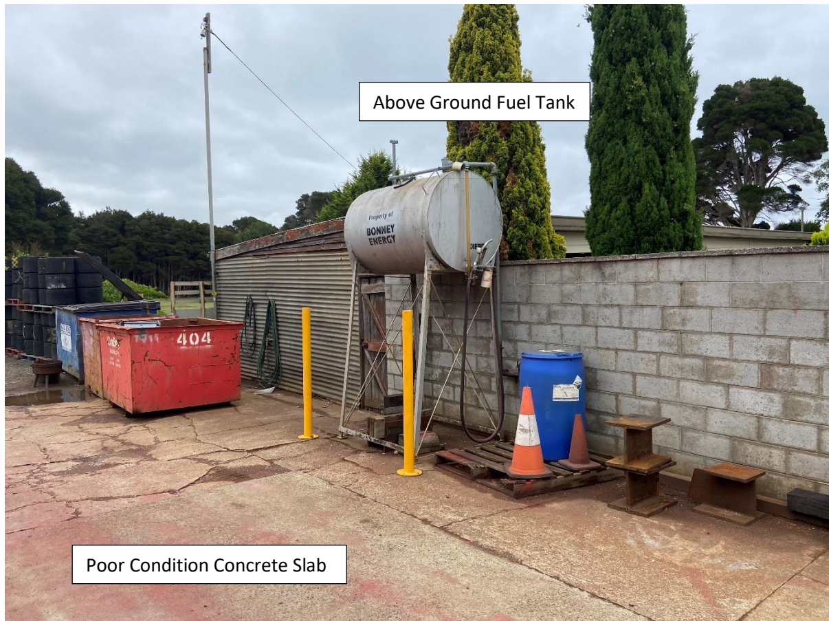
Figure 13: Fuel storage tank on broken concrete slab
