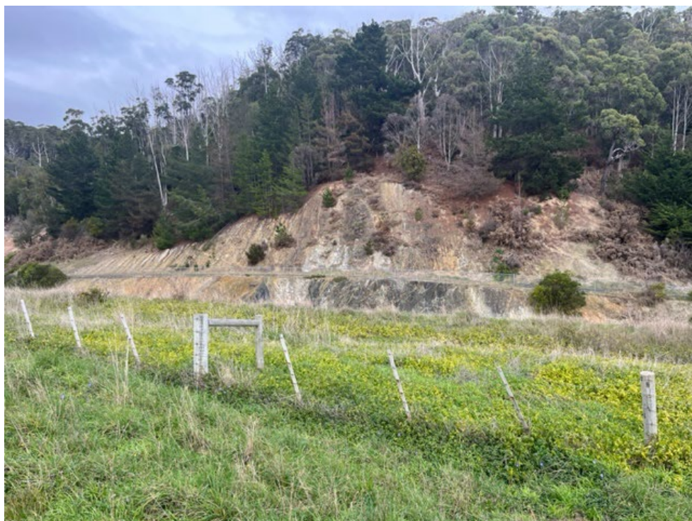
Figure 21 – View looking south from the top of Parcel 3. The Bass Highway formation is in significant cut at this location and well below the existing ground level of Parcel 3.
