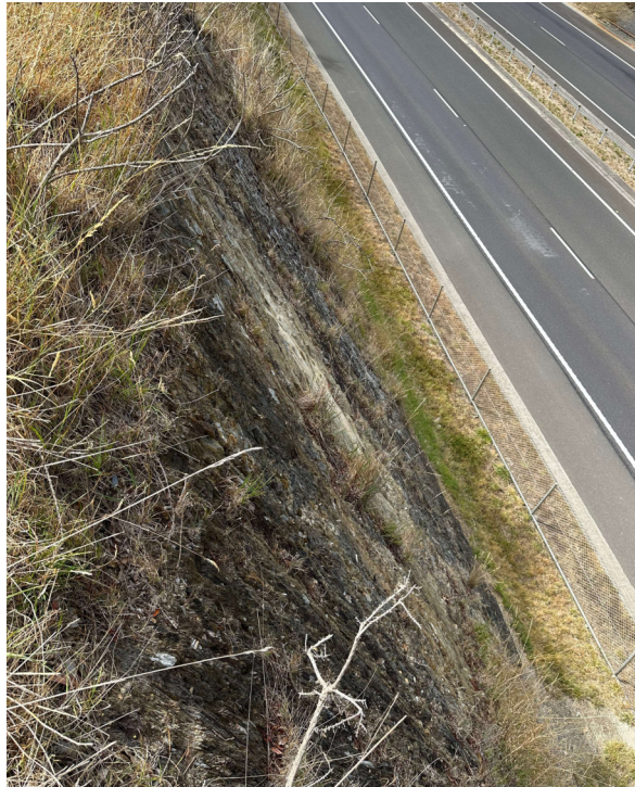
PLATE 3 - View of the road cut batter below Lot 3 along Bass Highway. Cut batter consists of insitu bedrock with a thin topsoil layer
