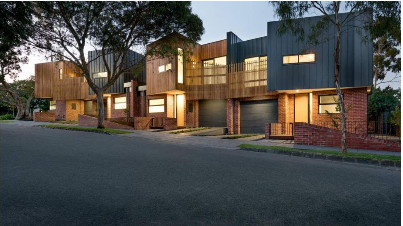
A simple materials palette. Alternating timber and metal cladding differentiates dwellings with consistent masonry podium.
