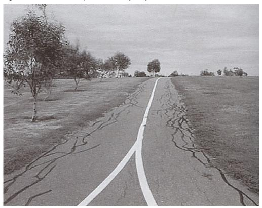
Figure C 2: Asphalt path requiring maintenance
