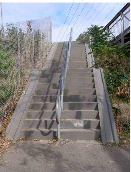
Figure 8.4: Example of a bicycle wheeling ramp
