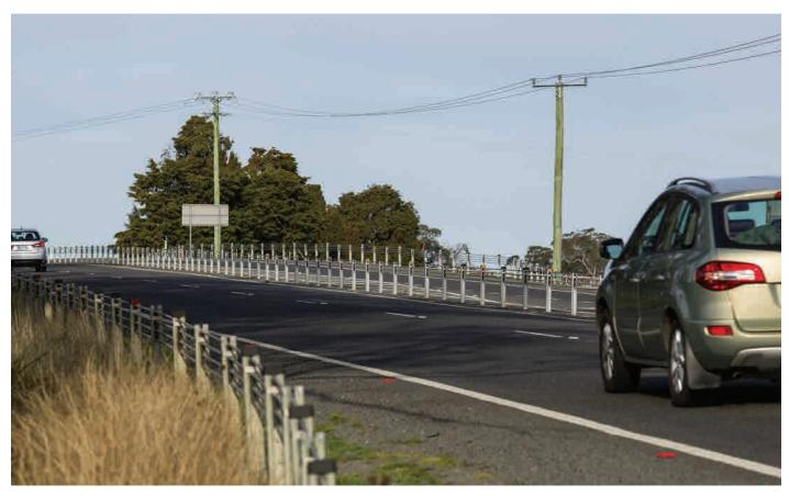
Flexible safety barriers provide full separation between vehicles travelling in opposing directions.
